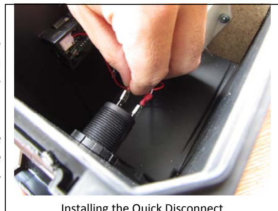
Installing the Quick Disconnect
