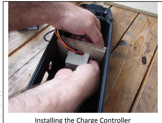
Installing the Charge Controller
